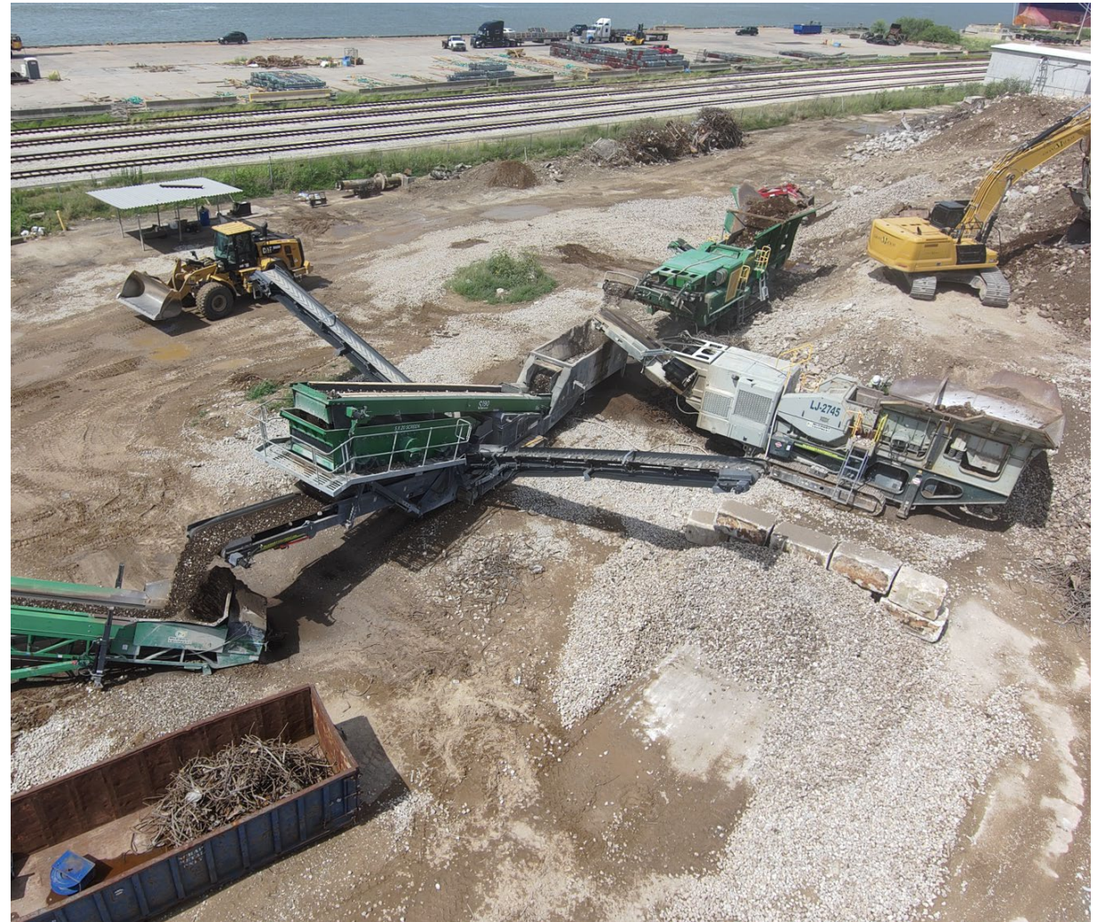
Showing Second Crusher Onsite
