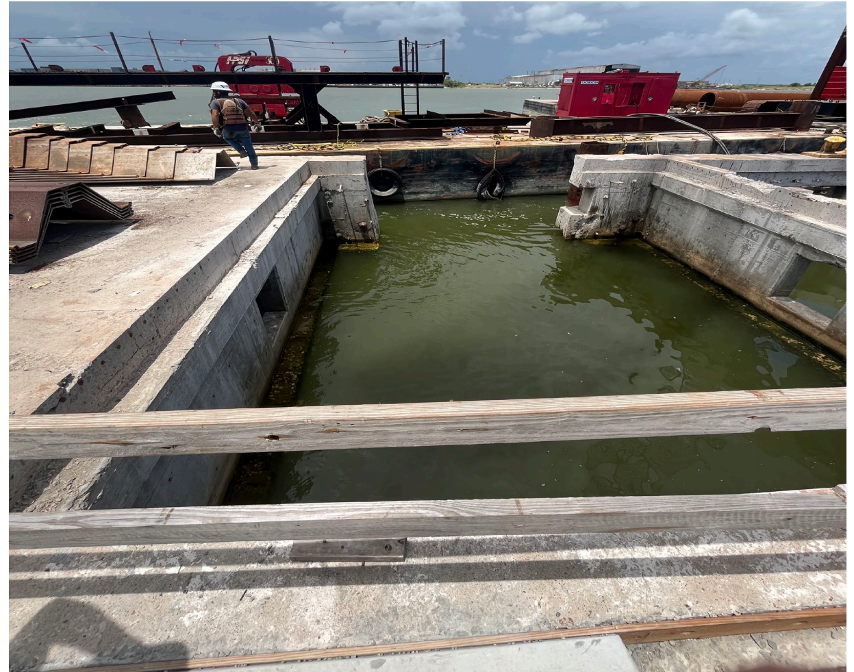
Pier 41 Return Wall Demolition
