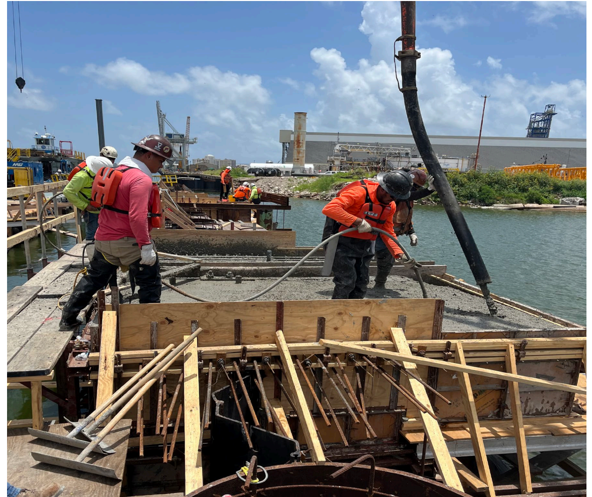
Concrete Placement for Fender Block
